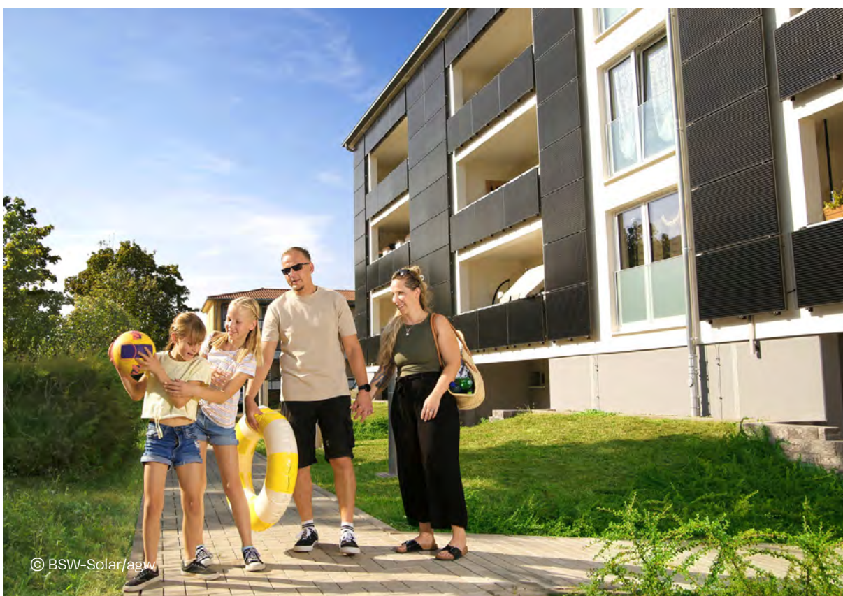
185 kW (114 kW roof, 71 kW façade) residential PV, Aschersleben, Germany. Project converting a prefabricated building into an almost energy-self-sufficient residential building.
