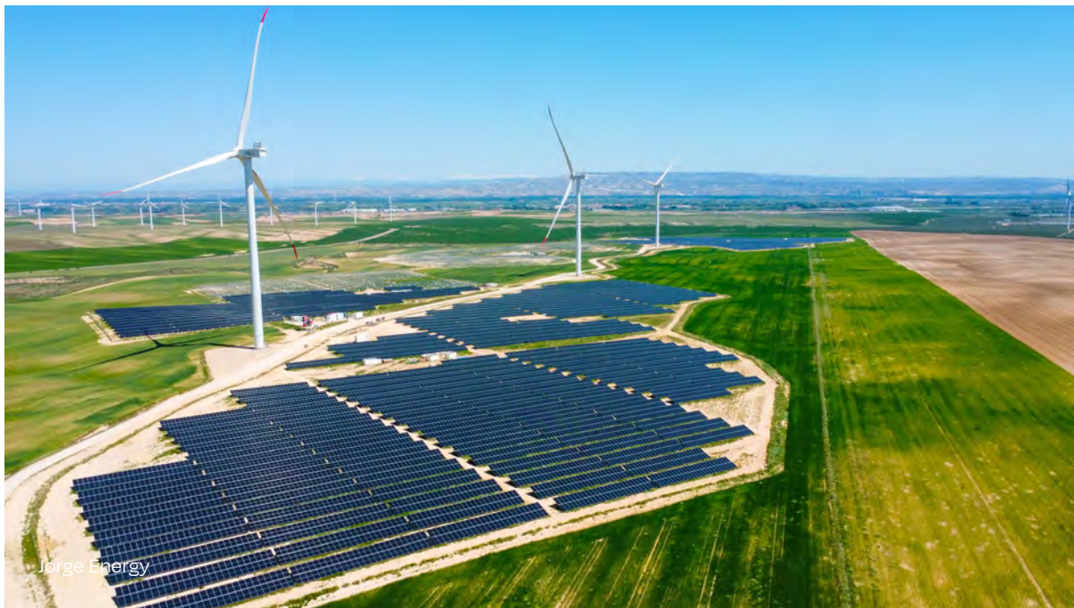
65 MW solar park by Jorge Energy and JinkoSolar in Zaragoza, Spain.
