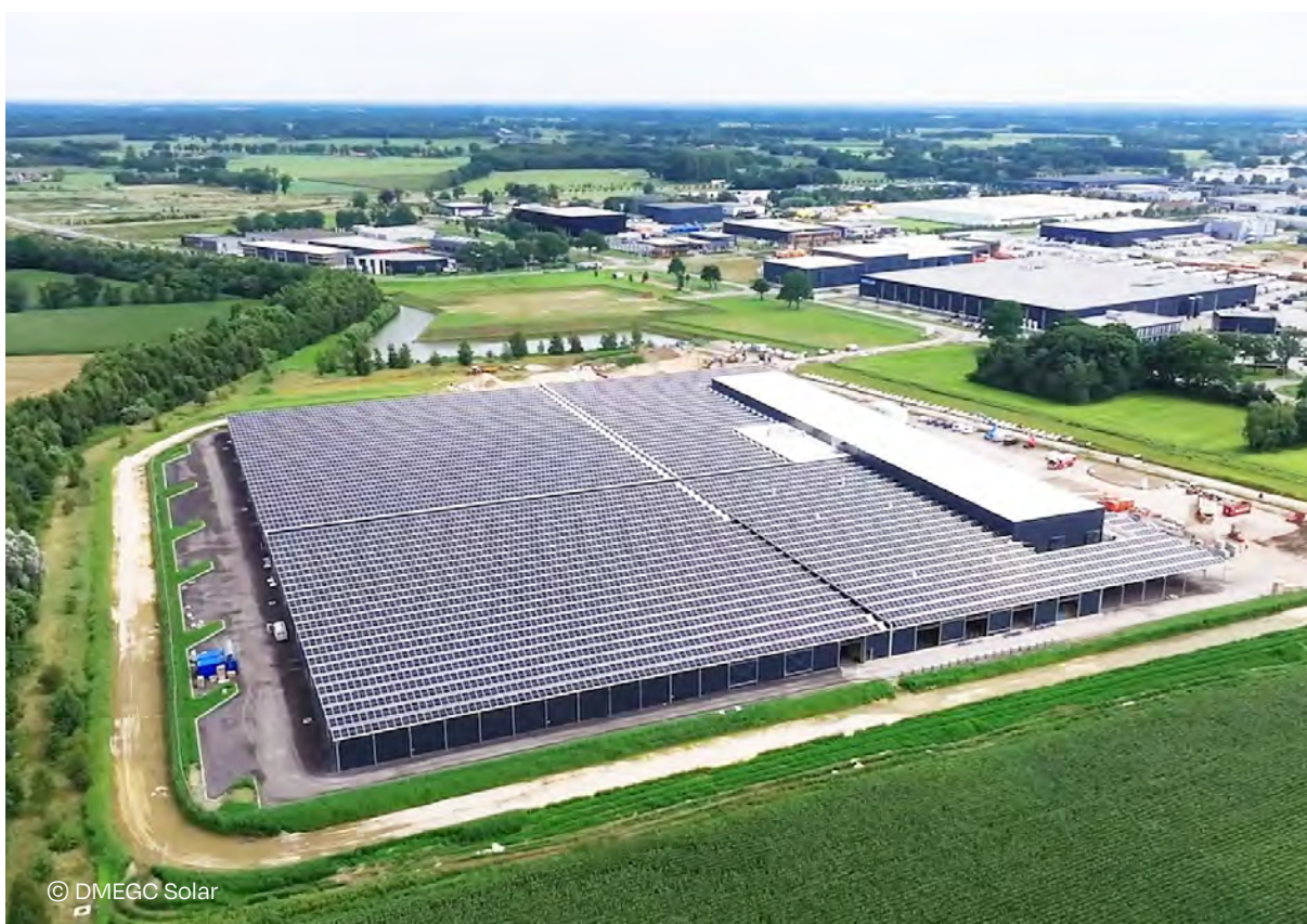
7.28 MW rooftop solar at Europe's largest camper and caravan center, Groenlo, the Netherlands.
