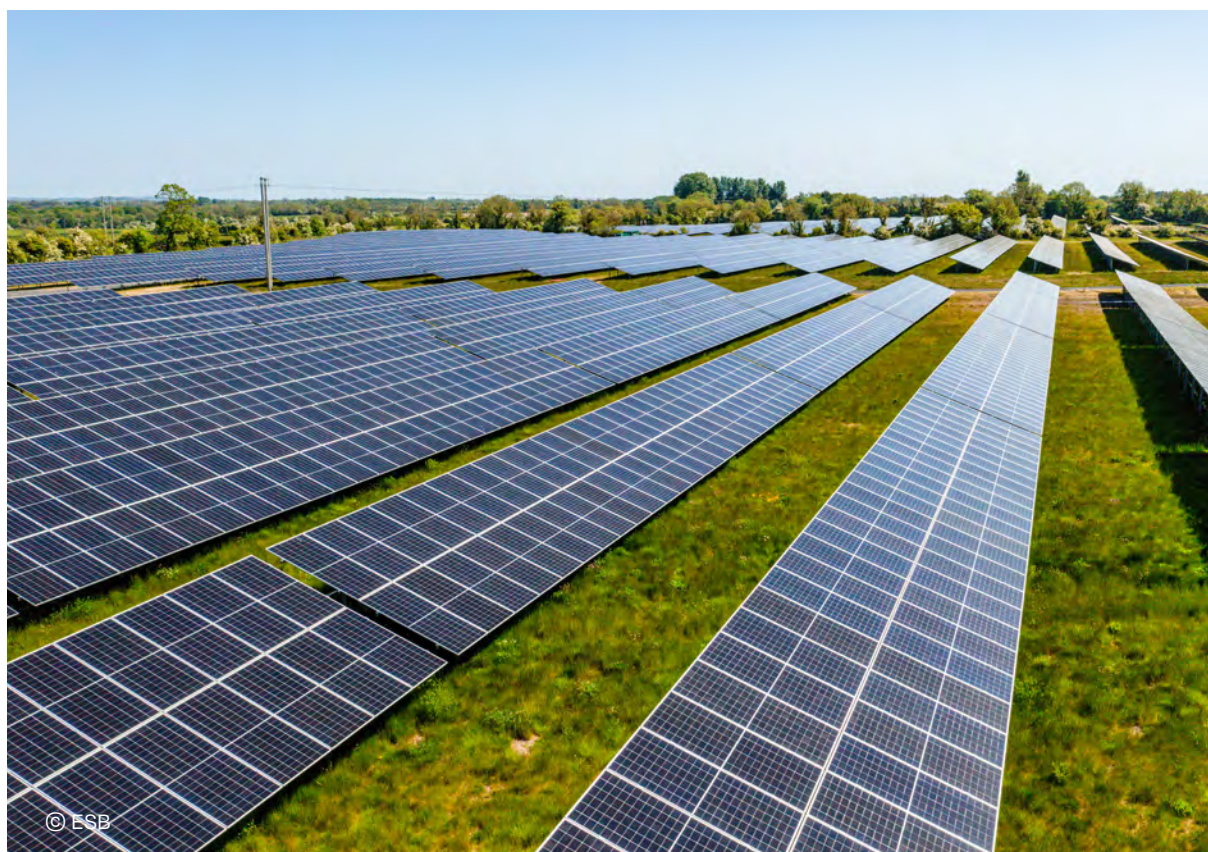
8 MW, Bullstown PV park, Ashbourne, Ireland
