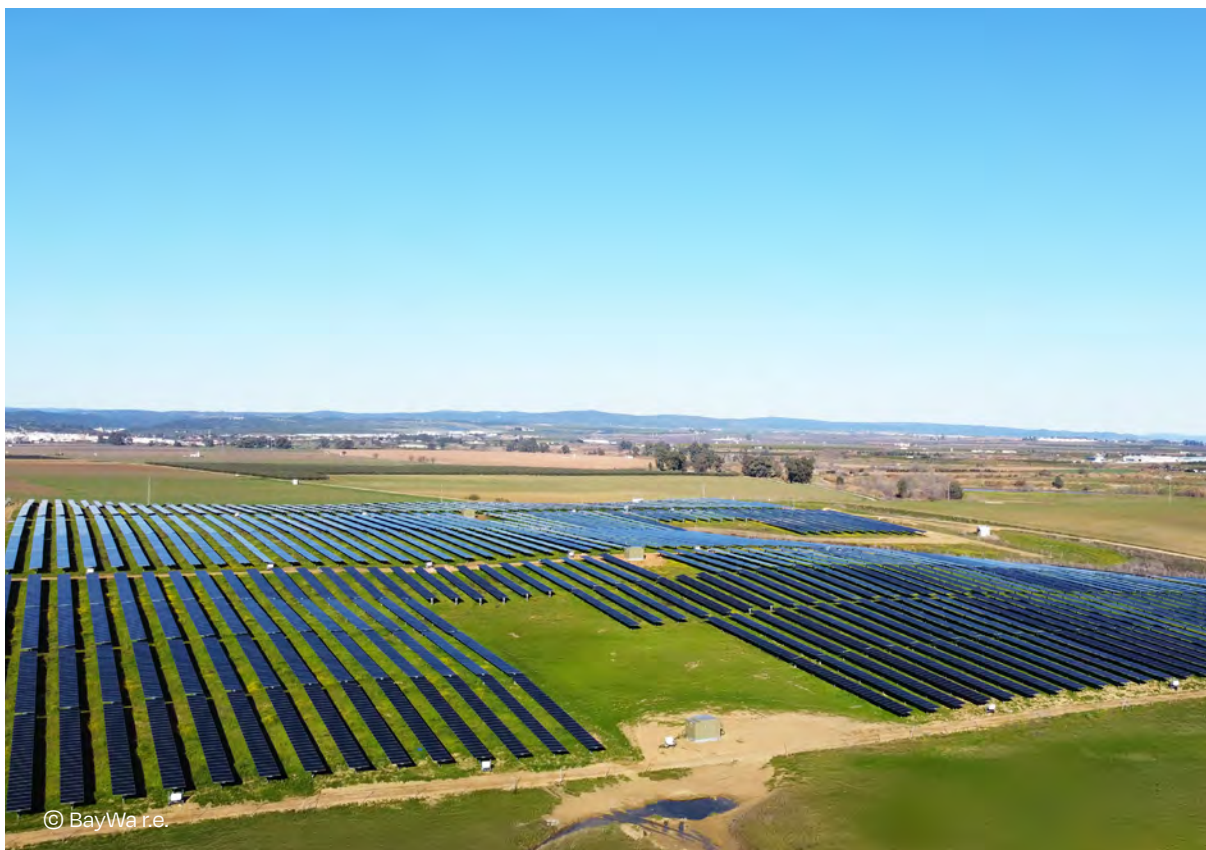
10 MW solar park in Chamorro, Spain.
