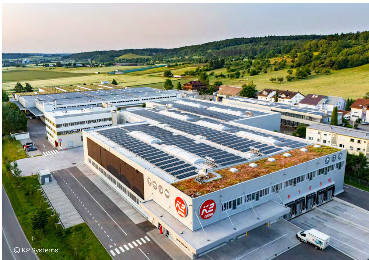
736 kW PV system on the rooftop and façade of K2 Systems' headquarters in Renningen, Germany.
