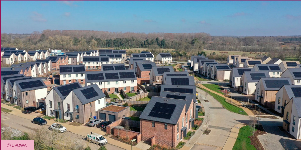
793 kW roof-integrated PV, 228 houses in a zero-carbon Eco-Town, Bicester, Oxfordshire, United Kingdom
