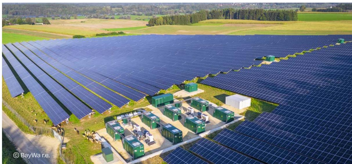
18.2 MW PV coupled with 6.2 MW / 20.7 MWh BESS, Deisenhausen, Germany
