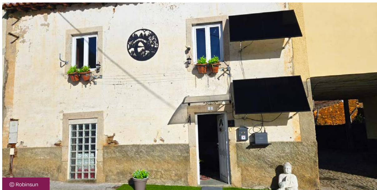
Façade plug-in solar, Mirandela, Portugal
