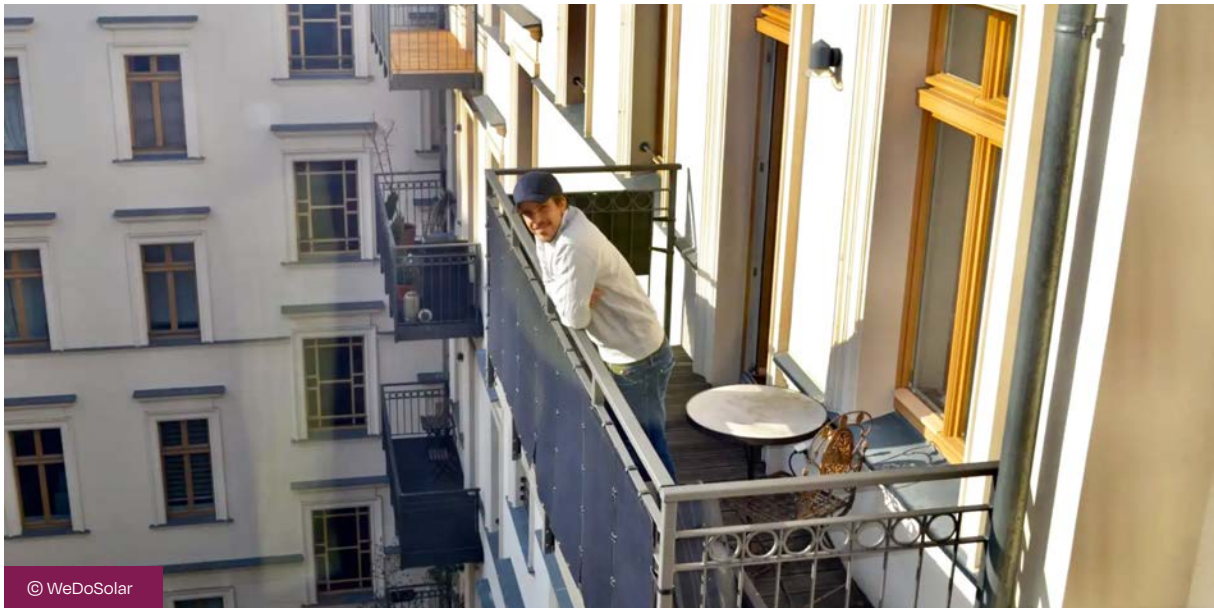
600 W plug-in PV, flexible solar panels installed on balcony, Berlin, Germany
