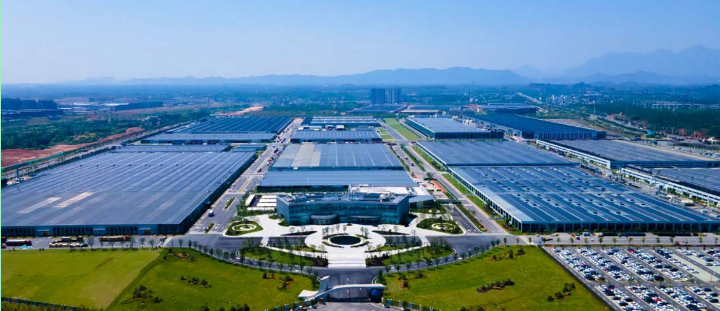
Shangrao module factory, powered by solar energy.
