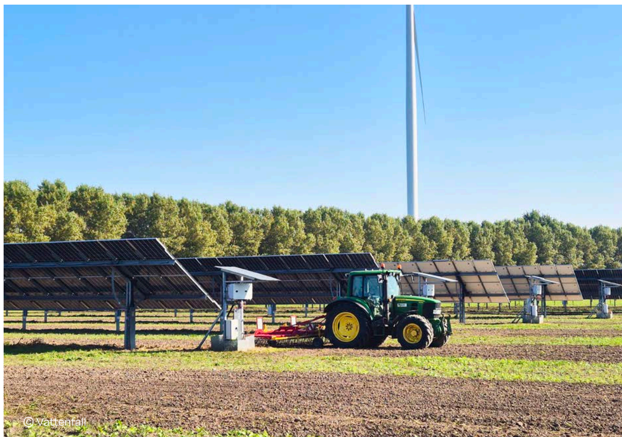
700 kW Symbizon solar PV plant, Flevoland, Netherlands
