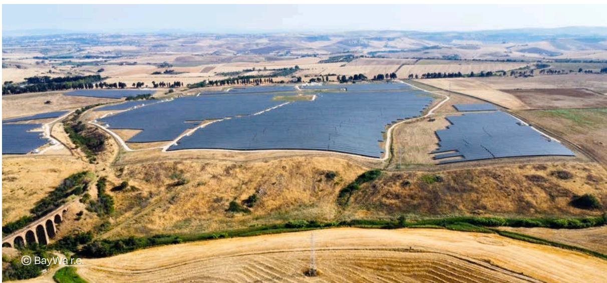
51.4 MW PV plant, Tarquinia, Italy
