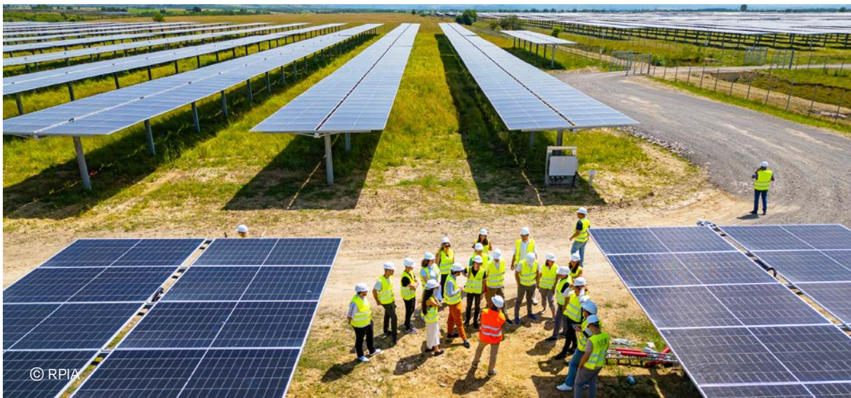
91 MW, Părău PV park, Solar Open Day 2024, Romania
