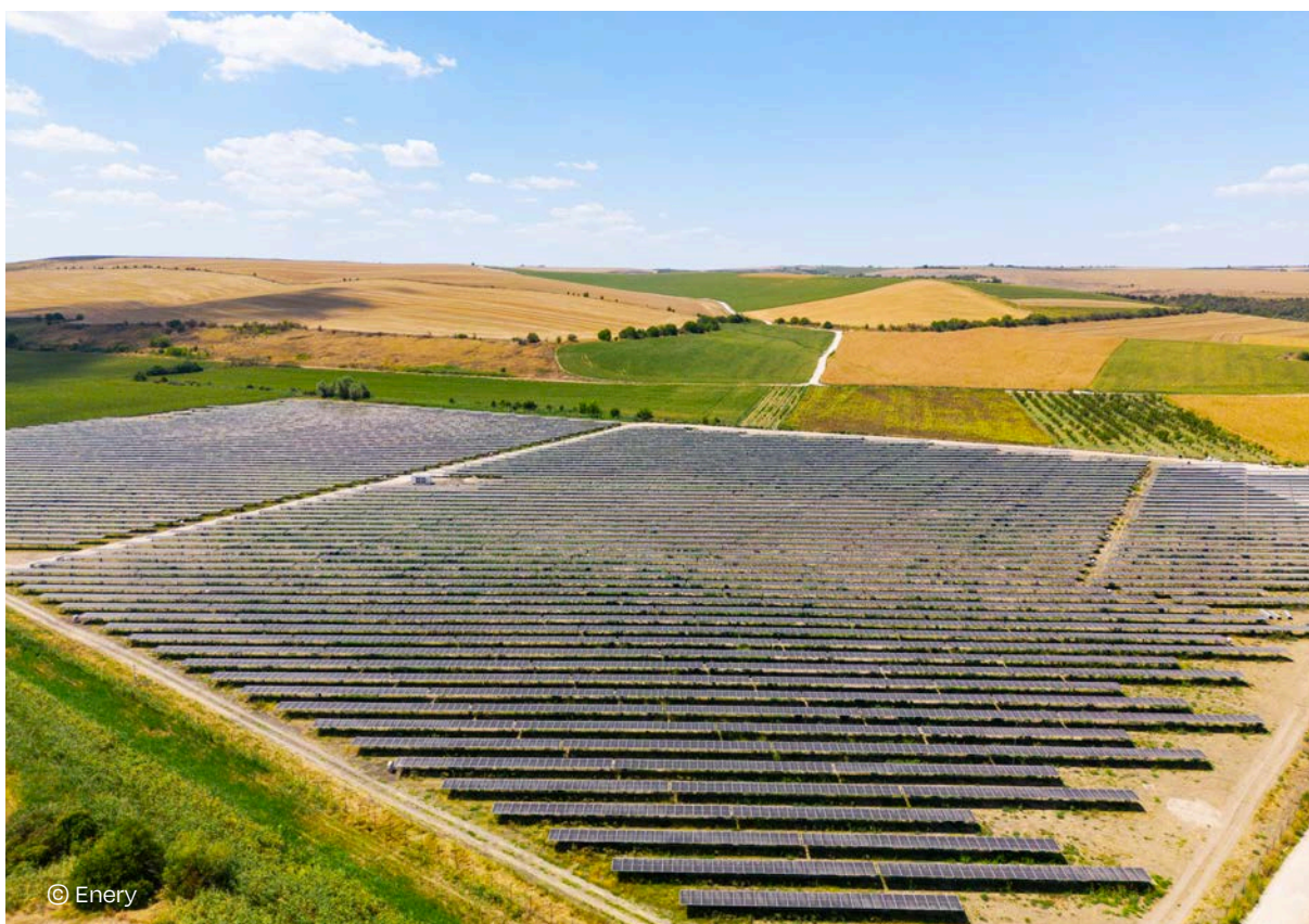
113 MW Tsenovo solar plant, inaugurated in October 2024, Bulgaria
