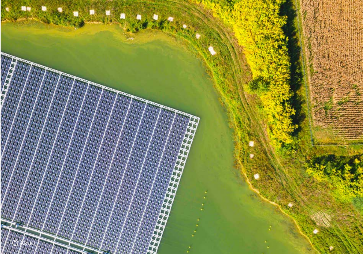
11 MW floating solar plant in Gouts, France
